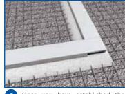
4 Once you have established the finish height and fall of the drain. Haunch the Ultra Drain Plus into place using either a concrete mix or sand and cement ensuring that the construction cover insert stays neatly fitted at all times in the Ultra Drain Plus base.
