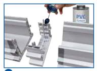
Use PVC glue in connecting the modular drain. Apply PVC glue on each part that you are joining and as per your drainage design fixing right angle corners and the outlets in their correct position.
