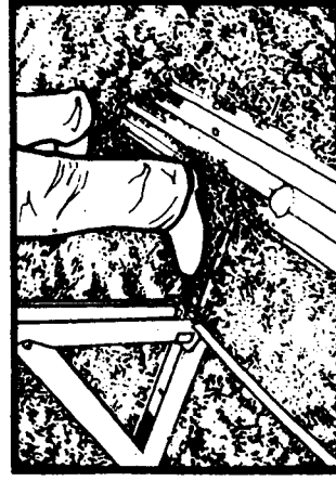
28 Your pool is now ready to concrete. Check vertical levels before concrete hardens and pour concrete into excavated holes to ground level.
