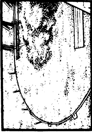
37 Slide the end rails into the connectors leaving approximately 32mm gap between them, and position with stakes so the rails conform to the radii marked out previously.
