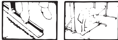
14 Repeat the procedure of Step 4 to 12. until all the pool frame construction assembly for your size pool are accounted for . At this stage temporarily install connectors and seats to aid in finding alignment and levels .
